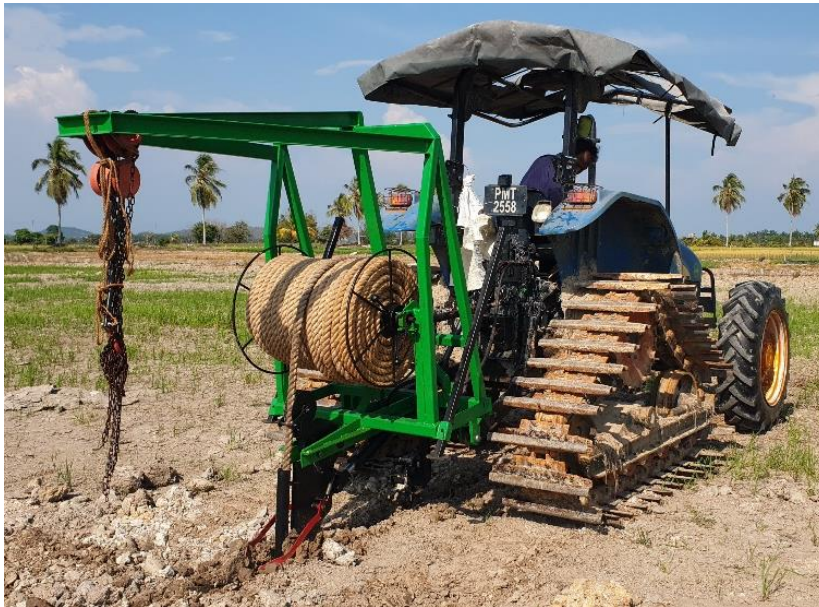
Figure 2: Mole plough with a rope applicator during a mole drain installation
